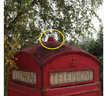
Femtocell on top of traditional phone box in East Garston
